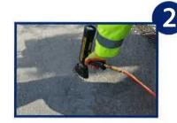
Using a suitable propane torch, remove any moisture present and preheat the area prior to treatment. Use a suitable primer on non asphaltic and aggregate rich surfaces.
