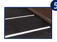
The HiFlex Tape should cool and harden within 5-10 minutes. When cooled, examine the tape and test by trying to lift. If areas do lift, repeat step 4.
