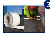
Remove the packaging and carefully place the HiFlex Tape onto the prepared surface with the glass coated top facing up. Position the tape as accurately as possible and cut to size.
