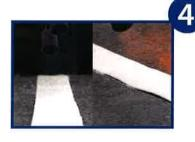
Heat the HiFlex Tape using a suitable propane torch keeping the flame approximately 20-40cm from the tape. Do not concentrate the heat in one area and heat with an even sweeping action. Heat until the tape starts bubbling and flowing into the road surface.
