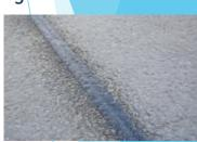
Clean application area thoroughly by removing all sand, dirt, chemicals and oily substances. Using a suitable propane torch, remove all moisture present (if any) and preheat the area prior to treatment.
